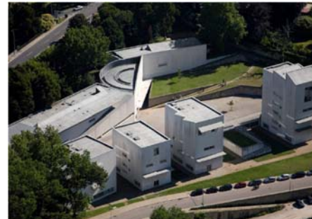
School of Architecture, Porto, Portugal – 1994
